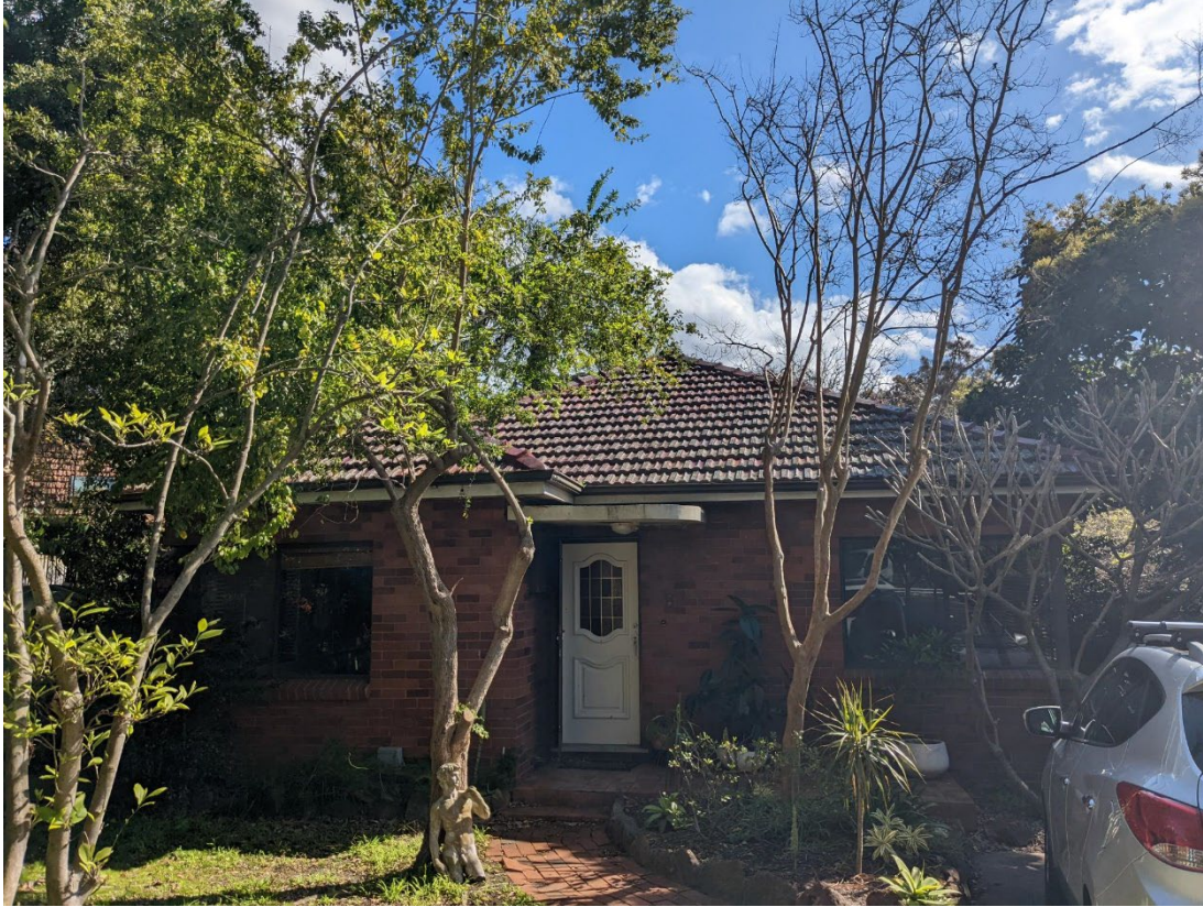
site viewed from Coneill Place
